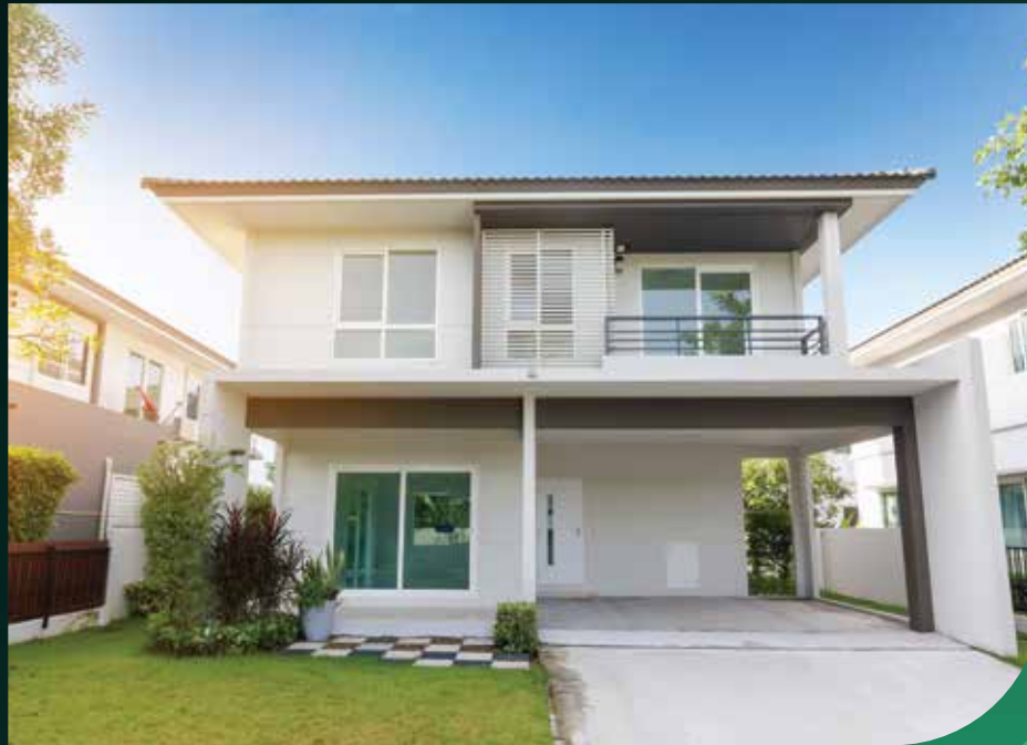
Individual Houses in industrial areas
